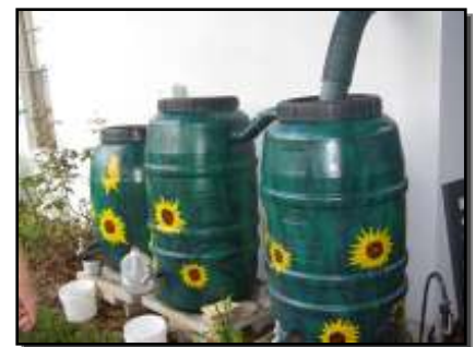
Multiple rain barrels used to collect rain water runoff from a roof.
