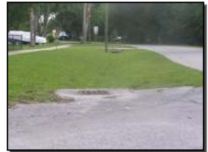
Example of a swale that is used for stormwater treatment in Pinellas County.
