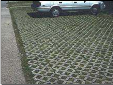
Example of pervious pavers installed in a parking lot.
