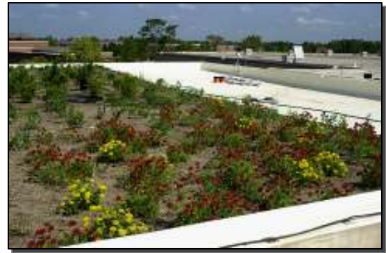
Green roof on top of the student union at the University of Central Florida in Orlando retains stormwater runoff and provides a mini-ecosystem.
