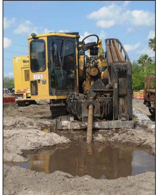
*Horizontal directional drilling installs pipeline segments under roadways, waterways and other key features to minimize impacts.*
