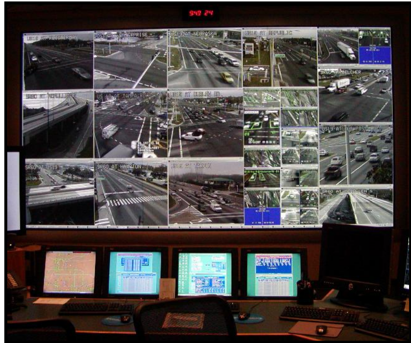
Figure 10: Pinellas County Traffic Control Center (TCC)
