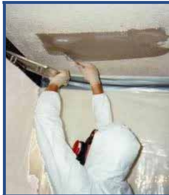
Licensed asbestos abatement worker removing asbestos-containing ceiling
