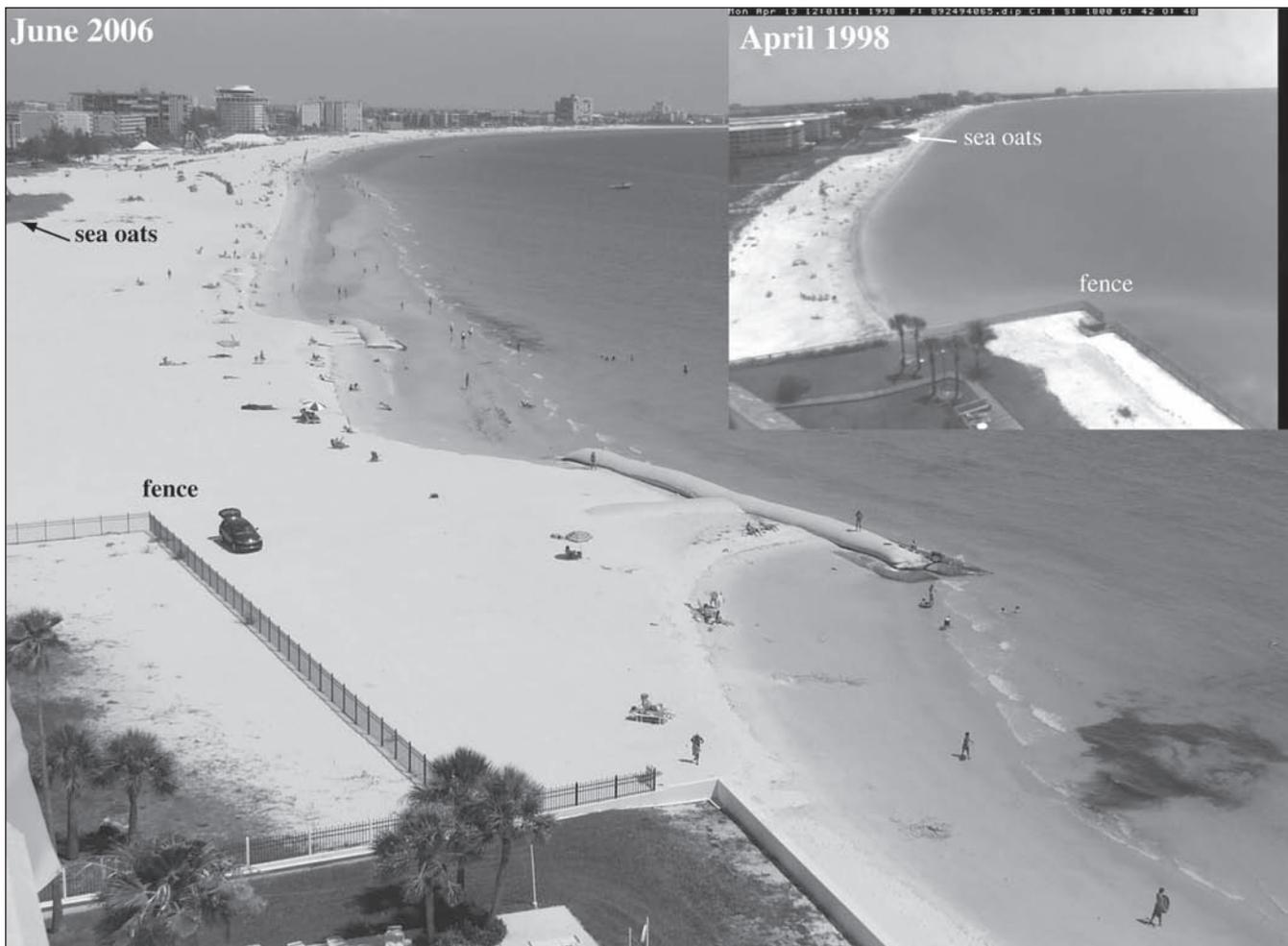
**Figure 8. Photos taken from the roof of one of the condominiums 22 months after the 1996 and 2004 nourishment projects. Note the wide beach stabilized by the T-groins in front of the fence and sea oats in 2006 as compared to 1998.**
