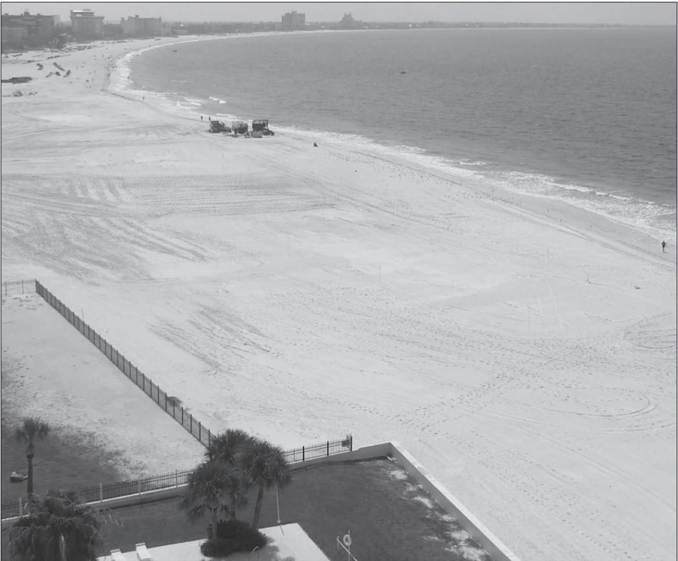
Figure 10. Recently renourished beach in September 2006 (compare to Figure 8). The T-groins are buried and are expected to become exposed gradually as the feeder beach erodes.
