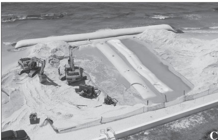
**Figure 7. Construction of the first T-head on: A) 19 April 2005, B) 16 June 2005, and C) 13 September 2005.**
