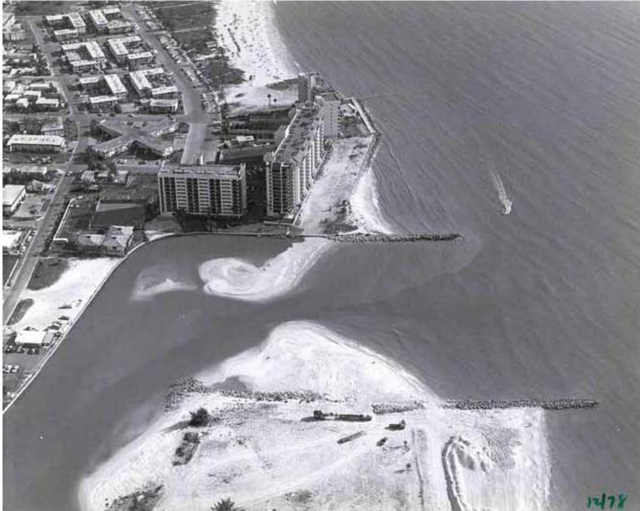
After this shoaling, the jetties were raised, lengthened, and sand tightened. A detached breakwater was added to the south jetty in 1986. During the 1960's, 70's, and 80's, Blind Pass was dredged nearly every 2 ½ years. By the 1990's, the downdrift erosion at Upham Beach was seemingly unstoppable. Due to the large volumes of sand trapped by Blind Pass, the only sediment source for the downdrift beach was nourishment. Blind Pass was last dredged in 2000 and the next dredging is planned for 2009.
