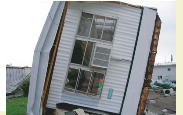
Tie-downs and hurricane straps can prevent your mobile home from coming loose.
