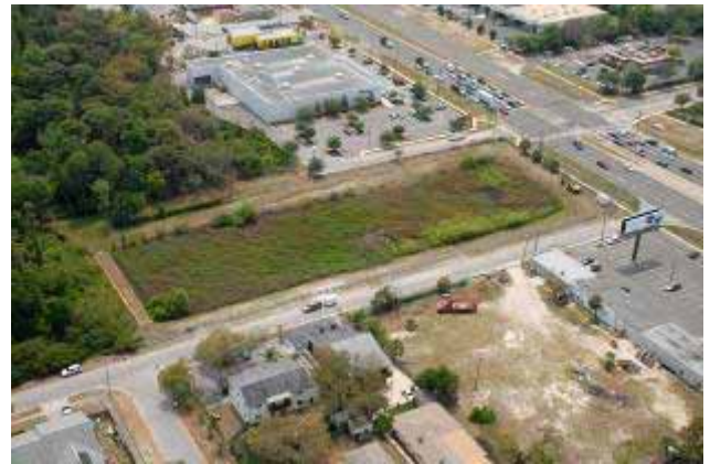
2. Looking southwest at Tarpon Area #6 prior to the construction phase.
