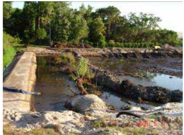
4. Looking south over the weir during dewatering and excavation process.
