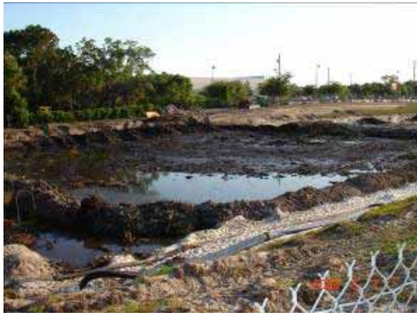
5. Looking southwest towards the Office Depot during dewatering and excavation process.
