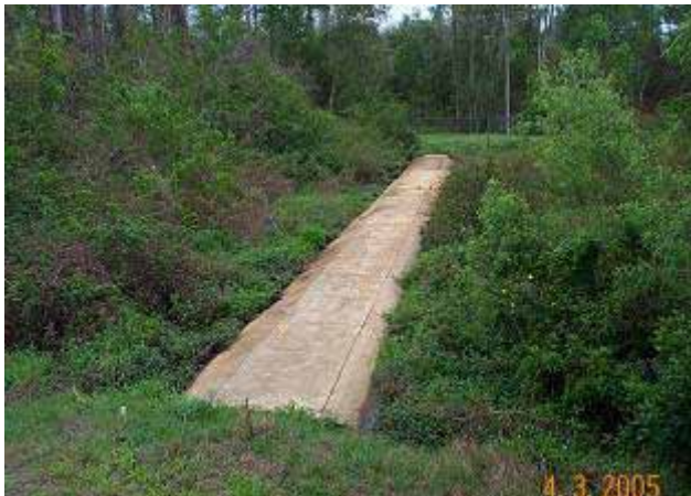
3. Looking south over the weir prior to the construction phase.
